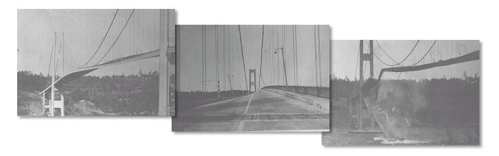
Perhaps an even more graphic illustration is the destruction of the Tacoma Narrows Bridge on November 7, 1940. That day there was a CONSTANT 40 mph wind blowing across the bridge. By chance, this was (obviously) precisely the resonant frequency of the bridge. The energy was absorbed and accumulated, causing the rhythmic bucking and swaying of the bridge for hours. The enormous steel girders eventually lost all structural integrity and the roadway collapsed.
