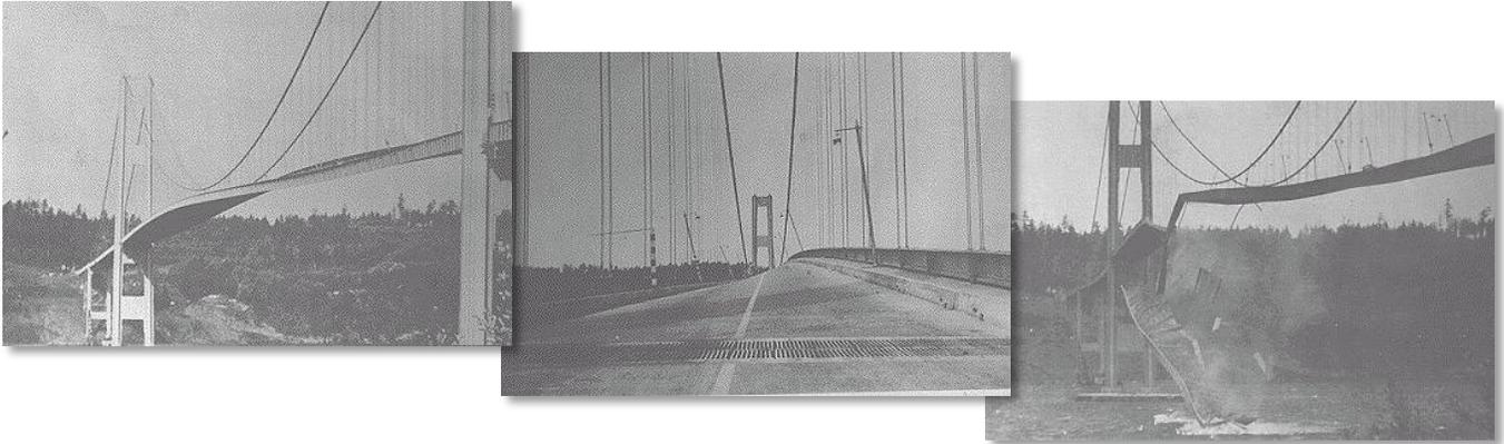
Perhaps an even more graphic illustration is the destruction of the Tacoma Narrows Bridge on November 7, 1940. That day there was a CONSTANT 40 mph wind blowing across the bridge. By chance, this was (obviously) precisely the resonant frequency of the bridge. The energy was absorbed and accumulated, causing the rhythmic bucking and swaying of the bridge for hours. The enormous steel girders eventually lost all structural integrity and the roadway collapsed.
